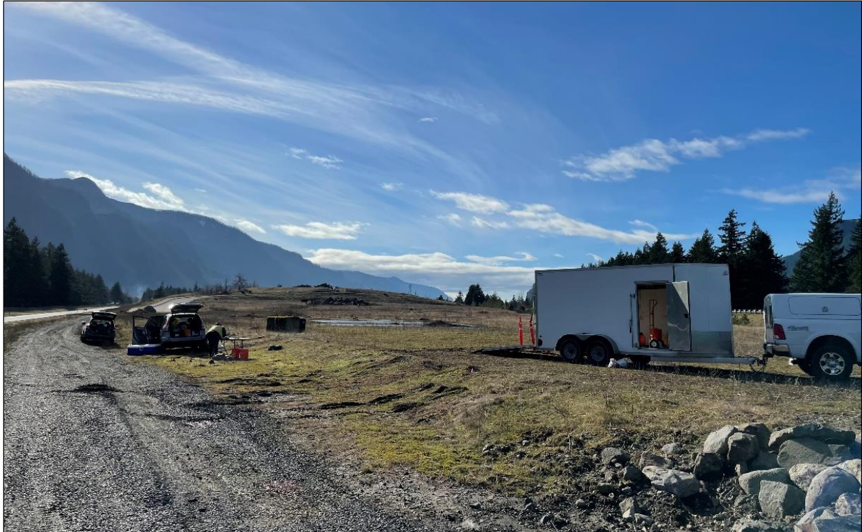
Figure 8. Overview of drilling work area, view west.
