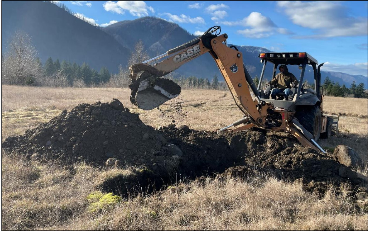
Figure 4. Excavation of TP-02, view southwest.
