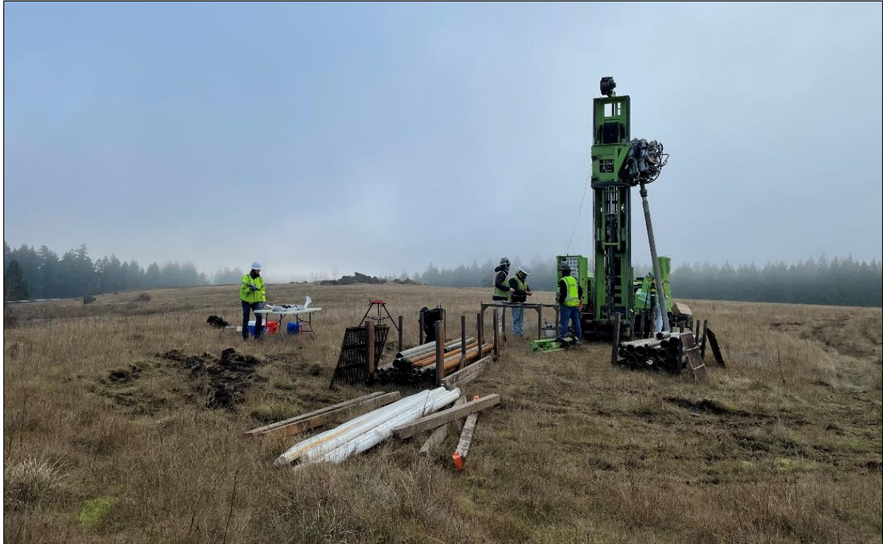
Figure 6. Overview of sonic drilling at B-06, view northeast.
