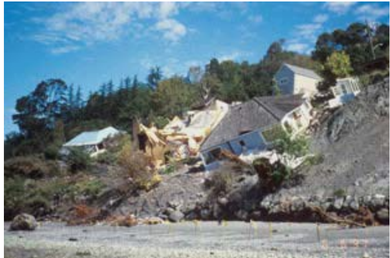
Homes destroyed in 1997 Perkins Lane landslide on Magnolia Bluff in Seattle
